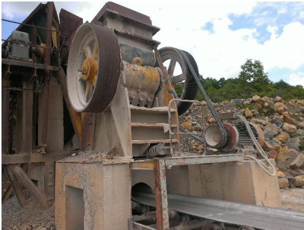
Fig. 3 General view of the crusher
