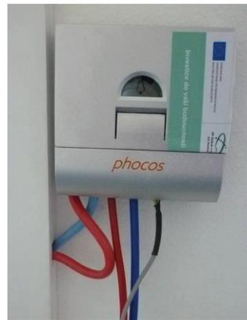
**Fig. 1.** The battery charging regulator of the solar power plant.
